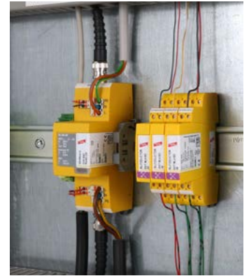
Space-saving and application-optimised 3in1 arrester DEHNvario
